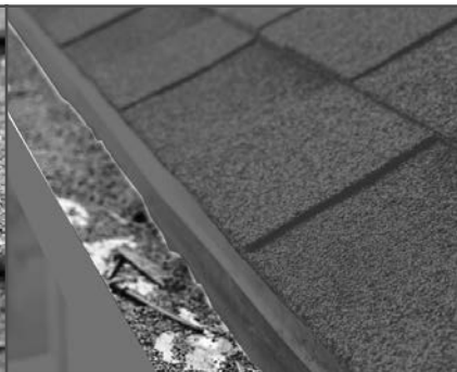
Granules in the gutter indicate shingle deterioration.
