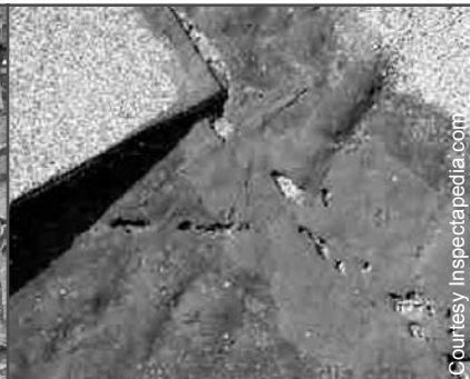
Roof cement loses its moisture content in time and cracks. Flashing, once installed, remains.
